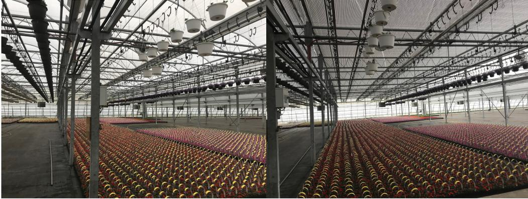
The main curtain project consisted of covering 28,080 square feet of roof area with Obscura XLS 18 Fire Break shade cloth
