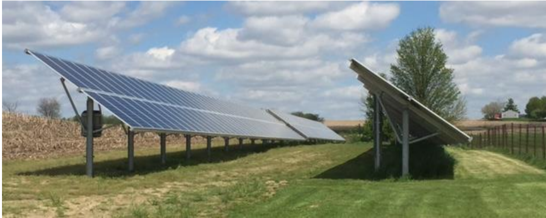
Figure 1 - The 75 kW solar energy system, positioned between a field and sheep pen.
