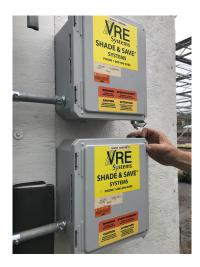
The boxes that were installed to control the power going into the curtains used relays and converters. The owner explained that this helps to tie them into an environment control system. He also stated that no maintenance is needed on the curtains themselves and the boxes require very minimal maintenance. In the ten years he has had curtains installed in sections of his greenhouse, he has enjoyed how user friendly they are and how well they work.
